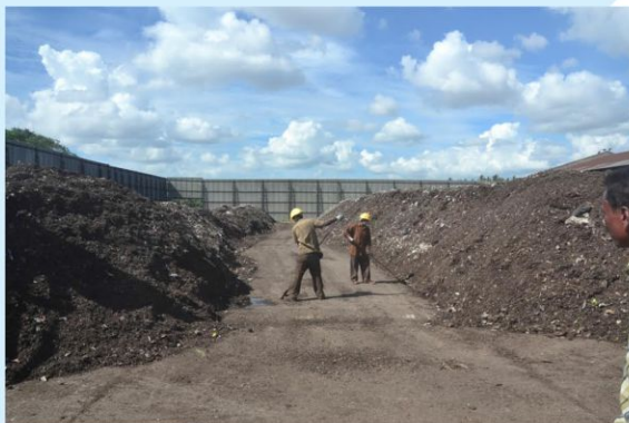
Remediation Under Process in Mysuru
