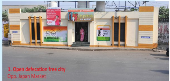
Public Toilet with All Facilities in Surat
